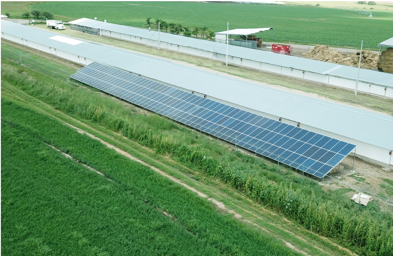
60KW Mexico PV Power Station This is a 60KW PV power station in Mexico, with 2 units
