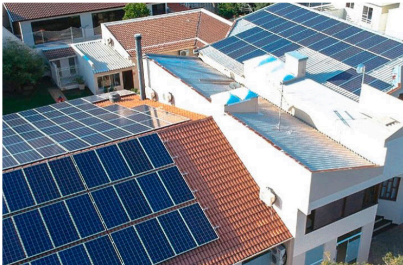
39KW Solar Plant in Curitiba Brazil 100 piece solar panels have been installed on the roof of a factory in Curitiba Brazil. Two NAC20K-DT inverters were deployed to power the facility
